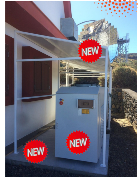
New chiller in place
