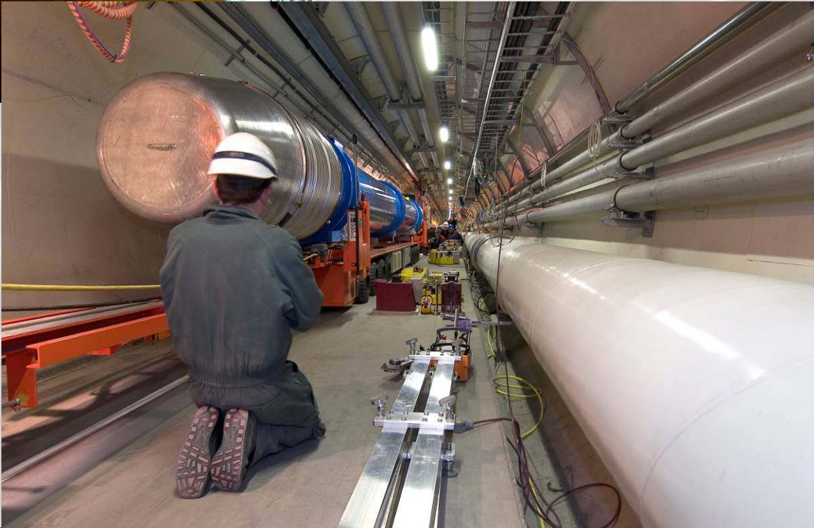
Installation of dipoles in the LHC ring
