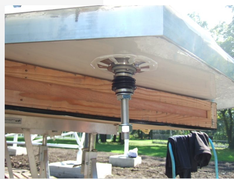
Mounting fix point on mirror
