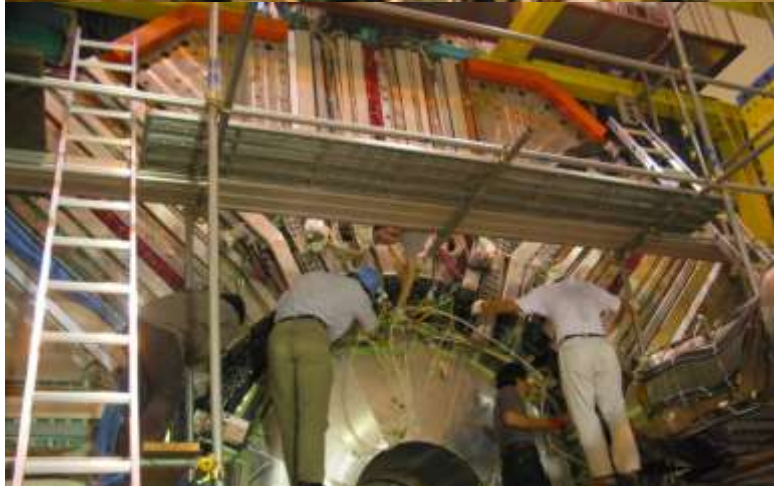
Connecting pipes and cables (ARICH,ECL)
