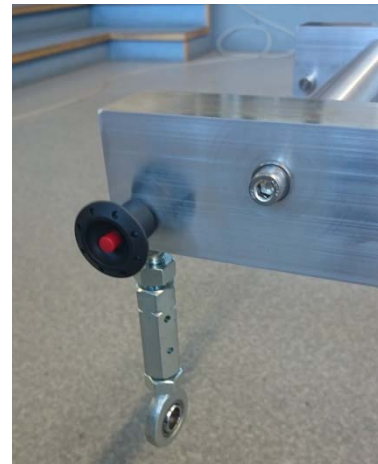
Fixation of cable trays
