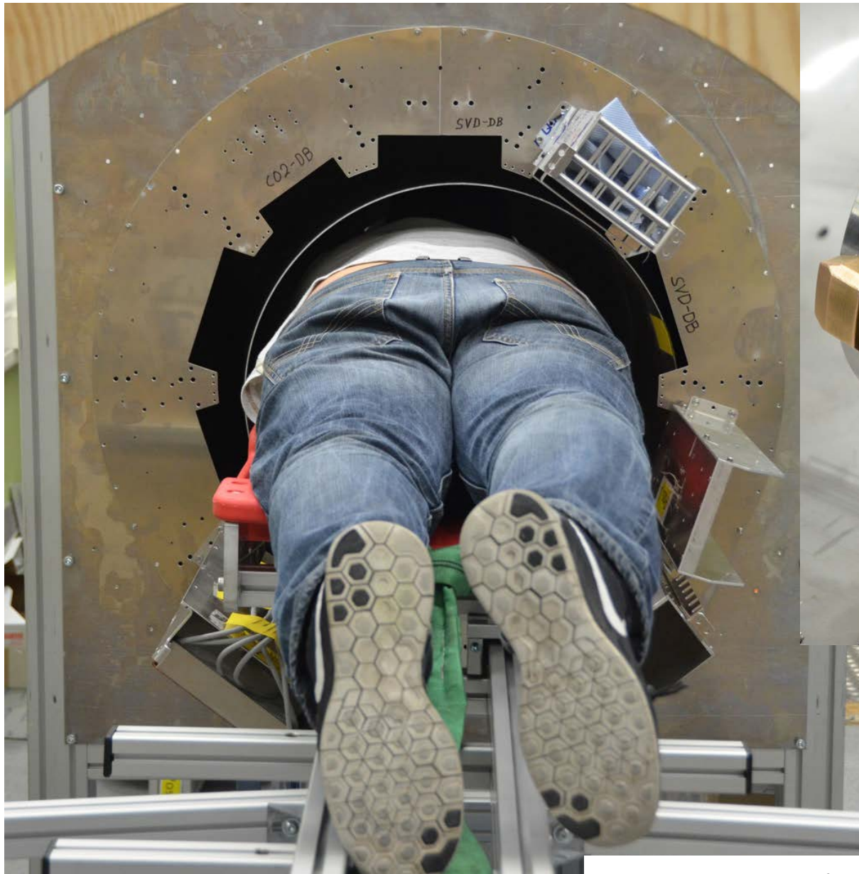
Installation of the bellows and connection of beam position monitors
