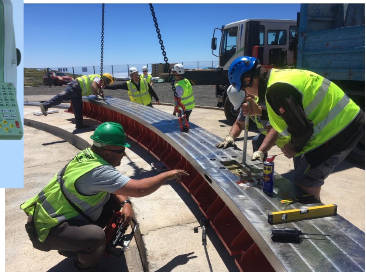
Sliding plates made of brass for temperature expansion
