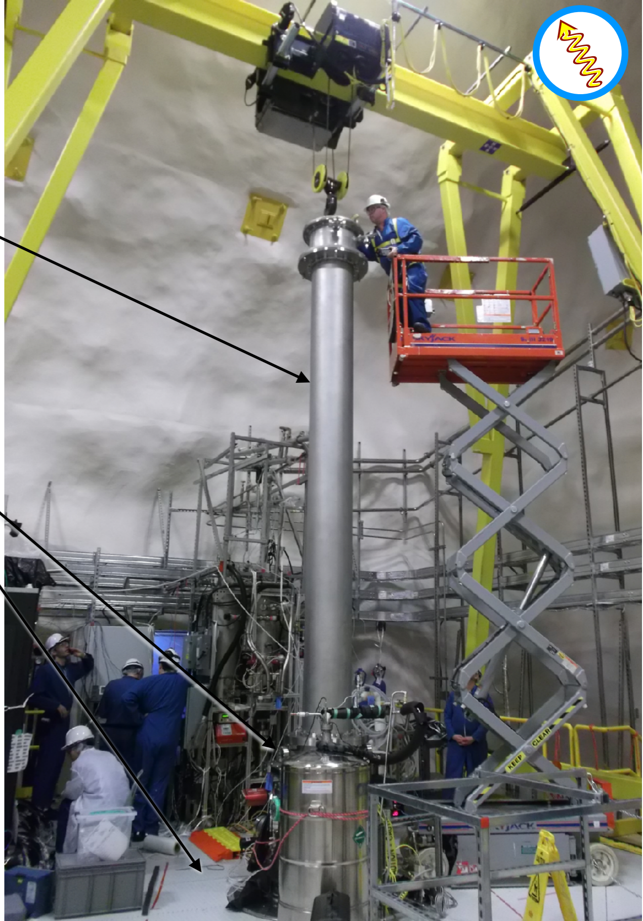
TPB deposition system being installed under air-tight conditions.
