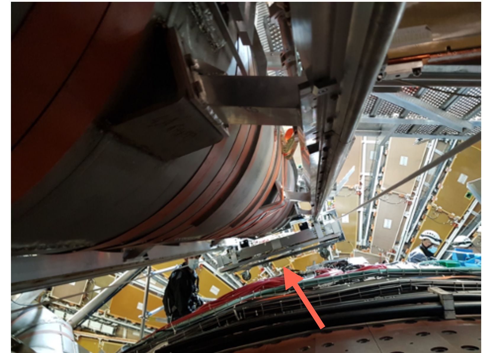
Chamber installed in sector A04
