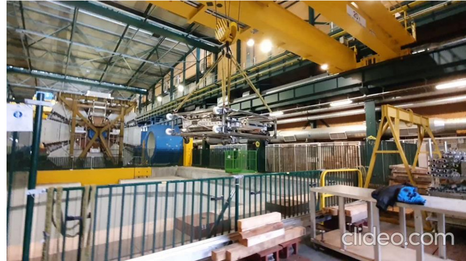
Installation of the station with two winches
