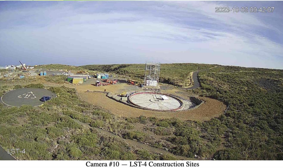
Camera #10 — LST-4 Construction Sites
