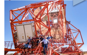
CT5 camera upgrade
