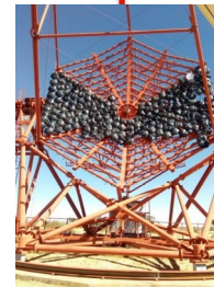
CT3 mirror refurbishment
