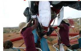
CT1-4 mirror refurbishment
